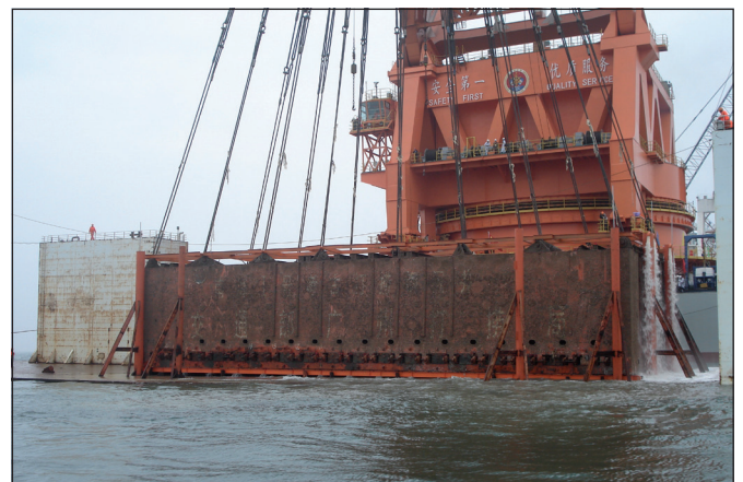
Figure 2: The protective container on the semi-submersible barge.
