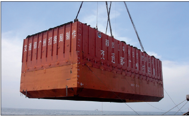
Figure 1: Steel open caisson.
