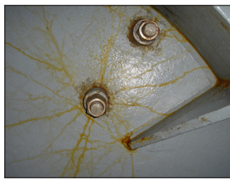
Figure 6: Bolts on outside of drum.
