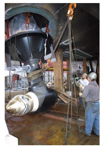
Figure 8 New ASD Unit Installation
