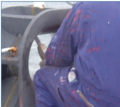
Coating removal using a needle scaler
